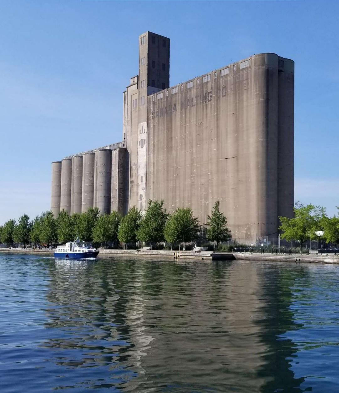
The south silos (1929) were designed by the John Metcalf Company and are an early example of the innovative explosion-resistant reinforced concrete grain elevator introduced in 1924. Toronto's earlier wooden grain elevators were all lost to fire
